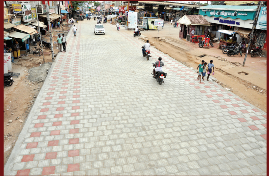
National Highways Authority of India - NH 210
