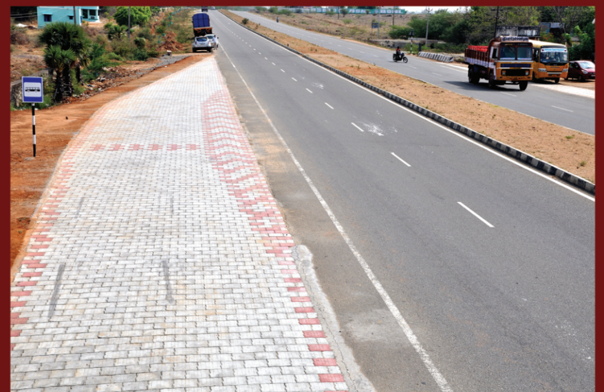
National Highways Authority of India - NH 7
