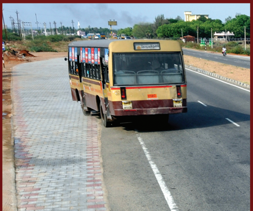
Bus bay - National Highways Authority of India - NH 7
